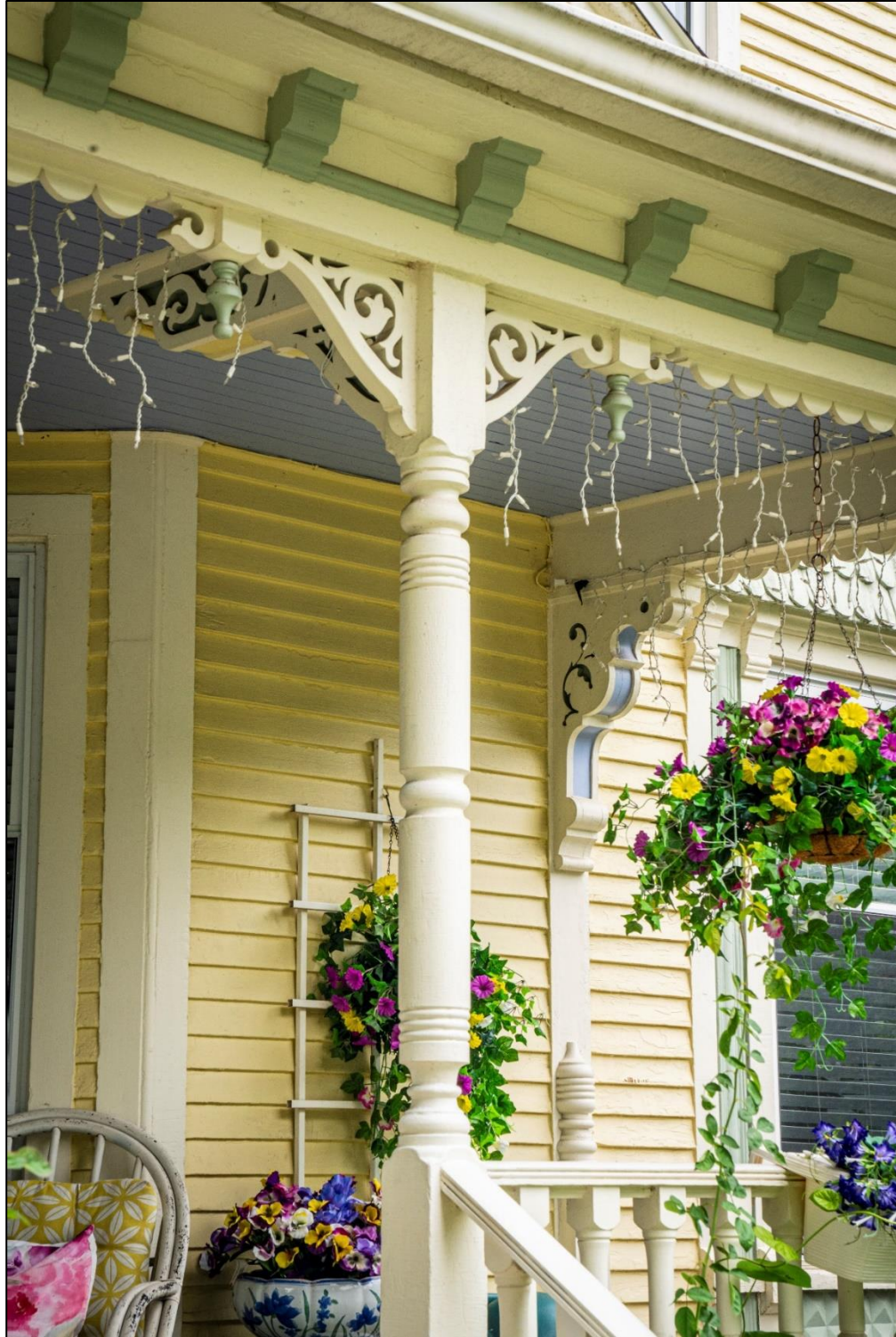
Restoration of Front Porch Award, Grand Rapids Historic Commission, March 2022 Photo Courtesy, Daniel Van Duinen
